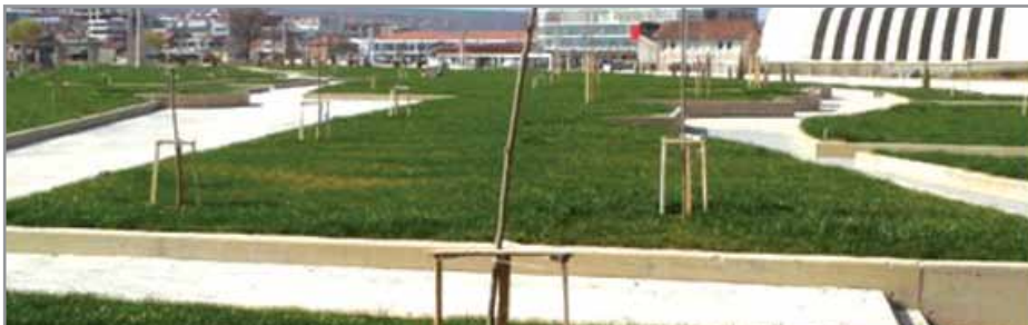
Construction views from "Rukolli" Company
